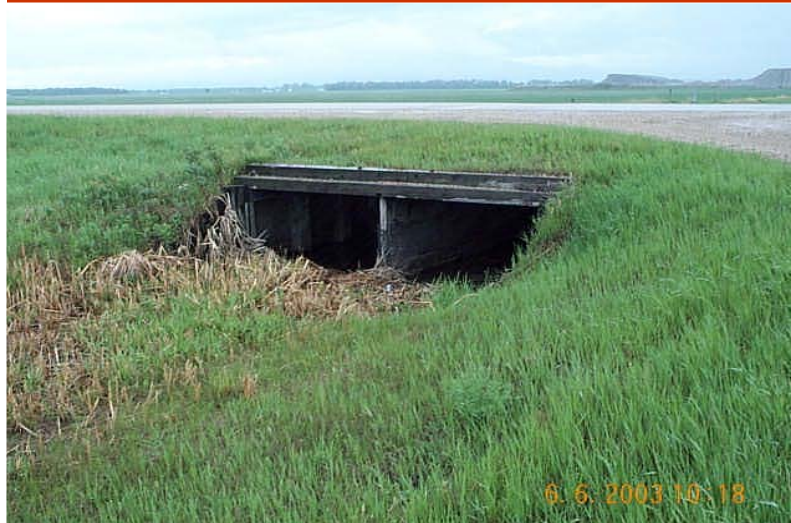
Figure 1: The Department includes large culverts in its bridge inventory
