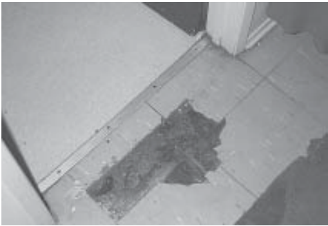
Excessively worn flooring is unsightly and contributes to sub-floor damage.
