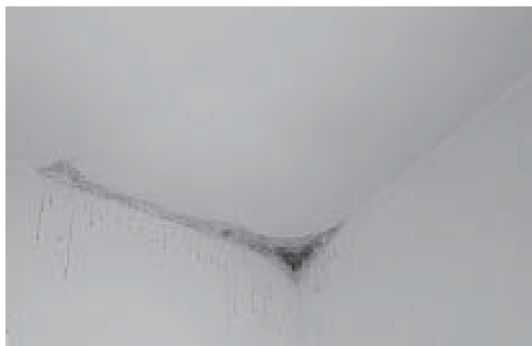
Moisture related damage and mould at ceiling can be caused by poor ventilation and/or insulation.
