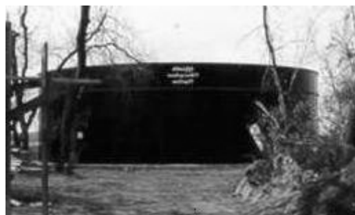
Steel tank manure storage facility
