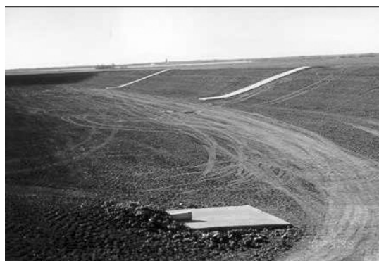
Earthen manure storage facility under construction
